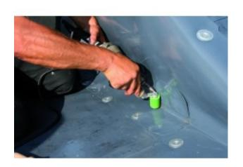
2 enclosed smooth-running ball bearings. Silicone roller. Bolted axis. Ergonomical wooden handle for maximum pressure. Bracket one-sided. For overlap welding. Ø 33 mm.
