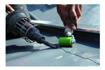
2 enclosed smooth-running ball bearings. Silicone roller. Bolted axis. Ergonomical wooden handle for maximum pressure. Bracket one-sided. For overlap welding. Ø 33 mm.
