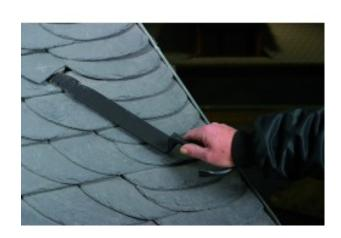
Traditional slate ripper. Welded. Made in steel.
