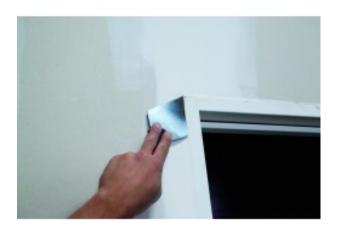
Stainless steel blade. Ideal to spread compound in inaccessible areas. Bi-material handle with metal head.
