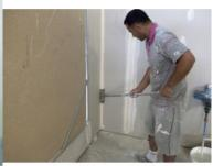
To tighten the drywall tape in the horizontal and vertical inside corners. 140 cm aluminium handle and stainless steel ball joint.
